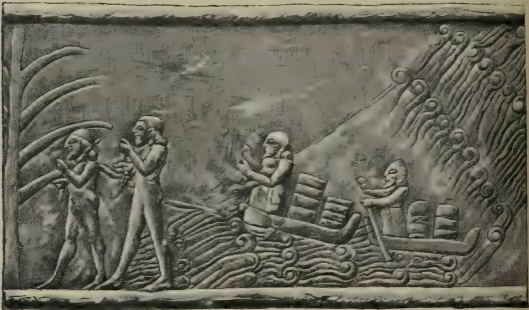
TRANSPORT OF BUILDING MATERIALS BY WATER. 2
